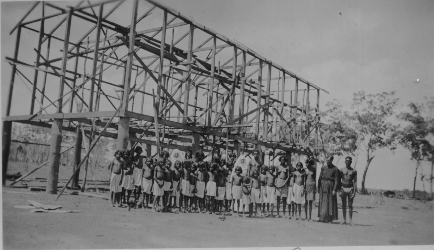
Shed built by J. D. Dabney and P. J. of natives
